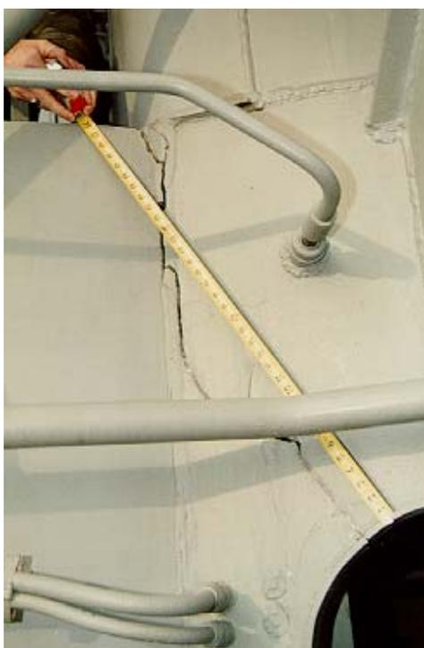
Figure 2. Crack Propagation
