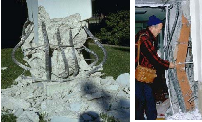
Figure 2. Buckling Failure of Reinforced Concrete Columns
